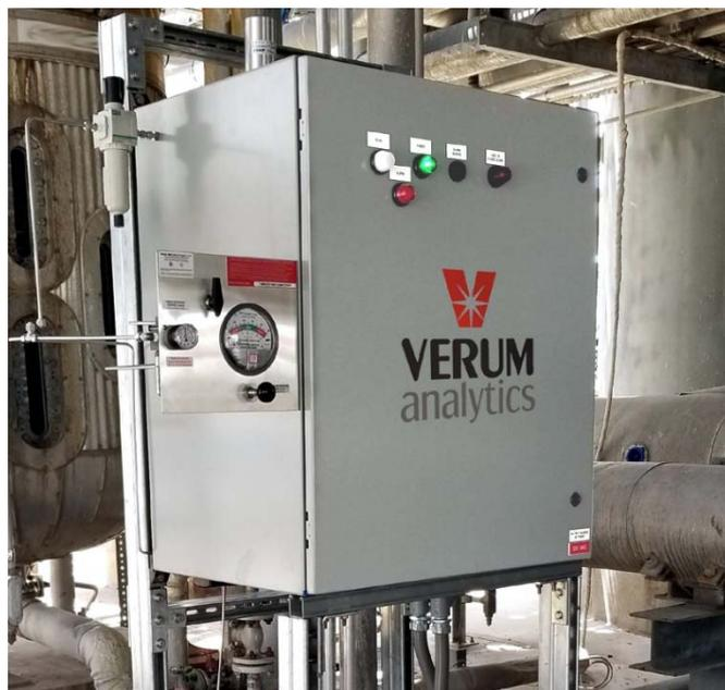
[Fig 5] Process NIR Analyzer (Verum Analytics IsoChem)
